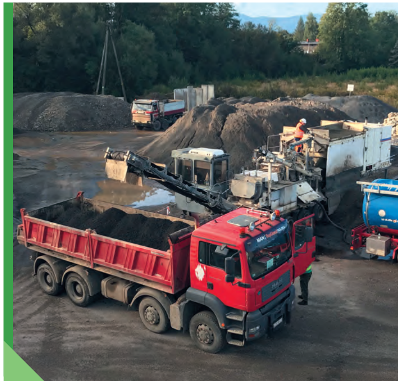
Fig. 5.1. Mobile GE mixing plant close to a construction site (photo Eurovia Polska S.A.)
