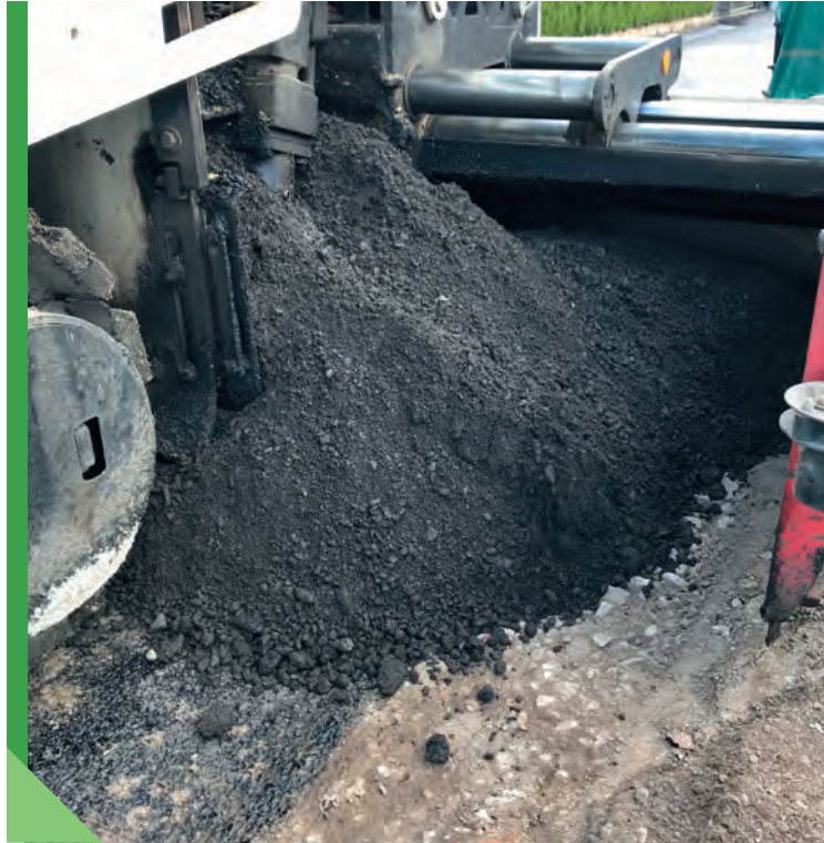
Fig. 5.2. GE mix in a spreader (photo Eurovia Polska S.A.)
