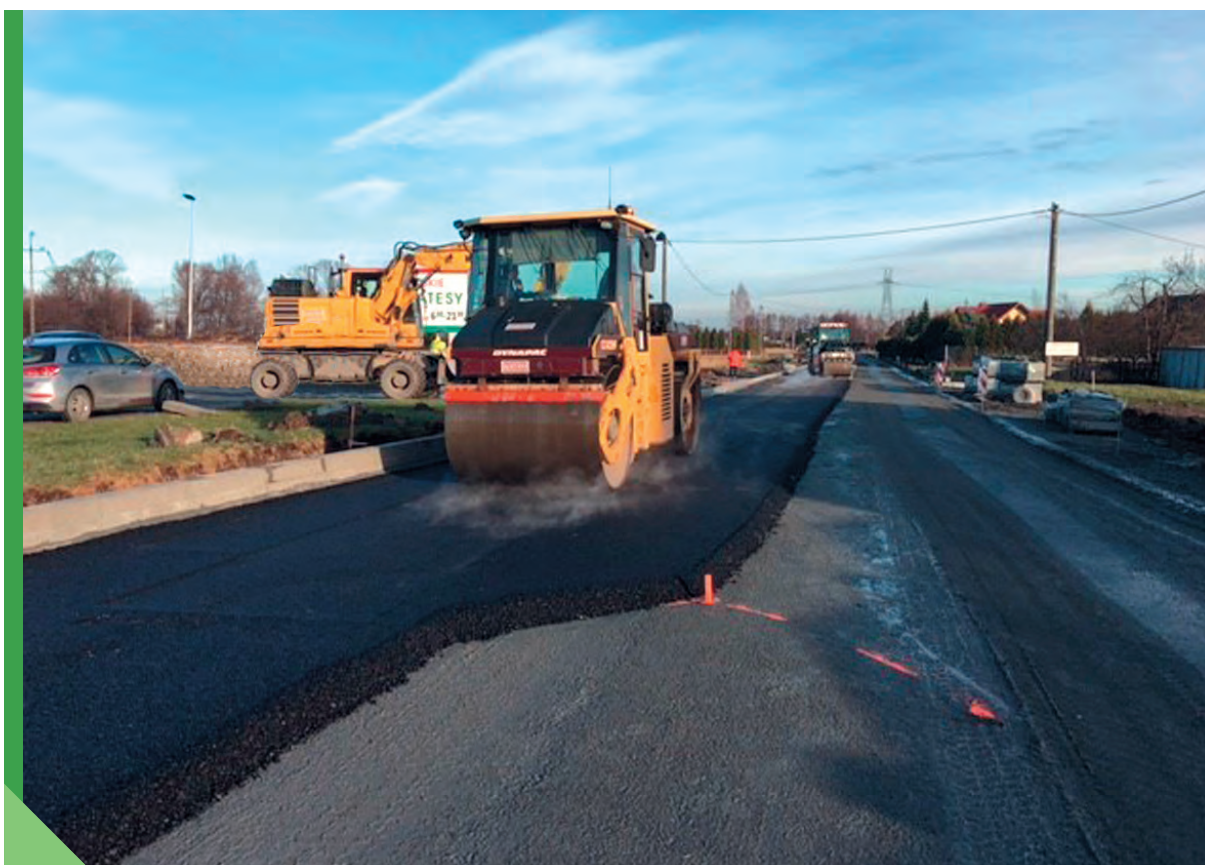
Fig. 3.18. Construction of an experimental road section using the ORBITON 45/80-80 HiMA WMA bitumen in 2021 [photo ORLEN Asfalt sp. z o.o.]
