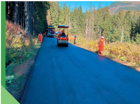
Fig. 6.10. Compacting pavement section made of the SMA 5 (photo P. Ostrowski, ORLEN Asphalt)
