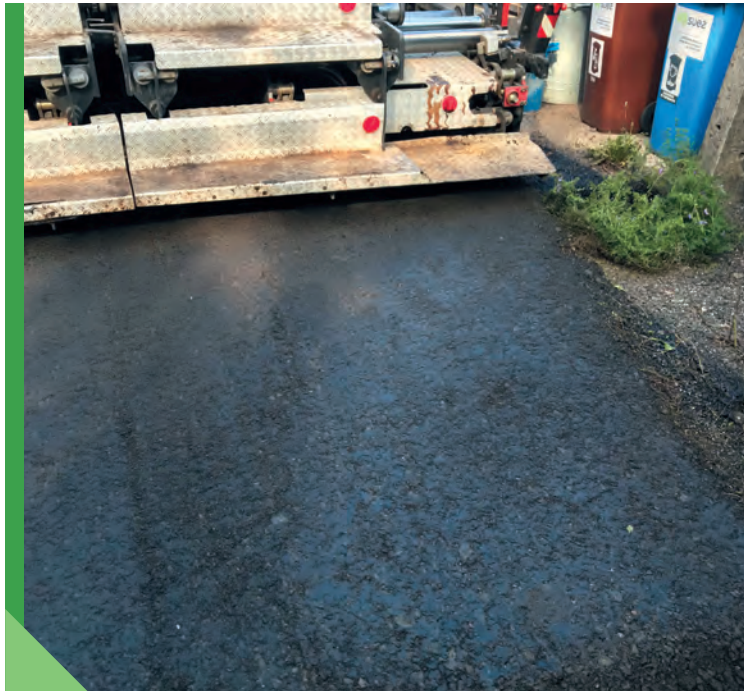
Fig. 5.3. GE mix right behind a spreader (photo Eurovia Polska S.A.)
