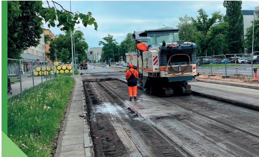
Fig. 4.1. Milling an asphalt pavement – selective milling of individual courses [photo P. Ostrowski, ORLEN Asfalt]
