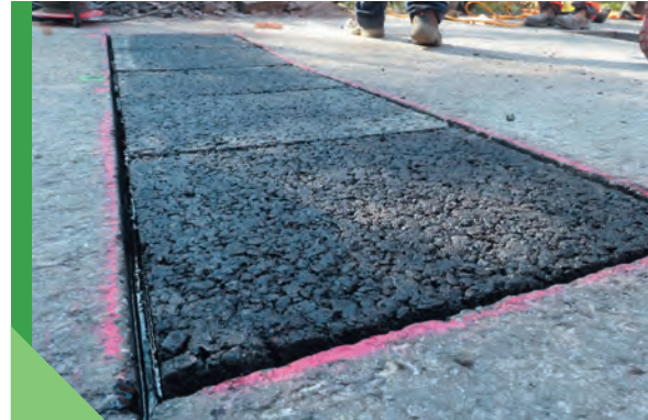
Fig. 6.9. One of the slabs (SMA16 mix) following installation in the pavement, prior to sealing (photo K. Błażejowski, ORLEN Asphalt)
