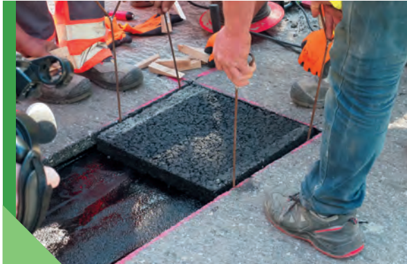
Fig. 6.8. Placing the slabs in autumn 2018 by OAT sp. z o.o. (photo K. Błażejowski, ORLEN Asphalt)
