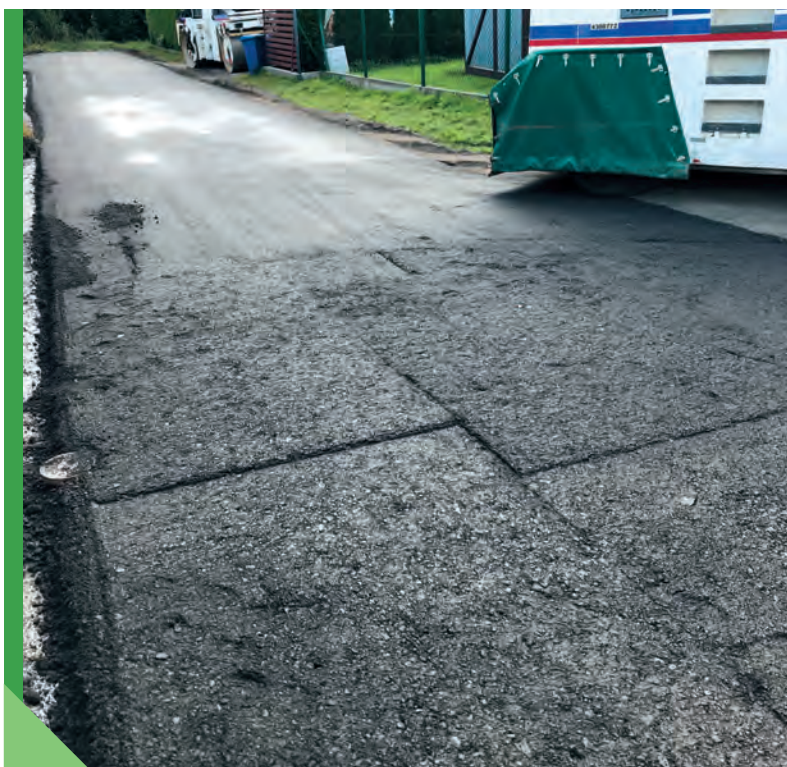
Fig. 5.4. GE mix during compacting (photo Eurovia Polska S.A.)
