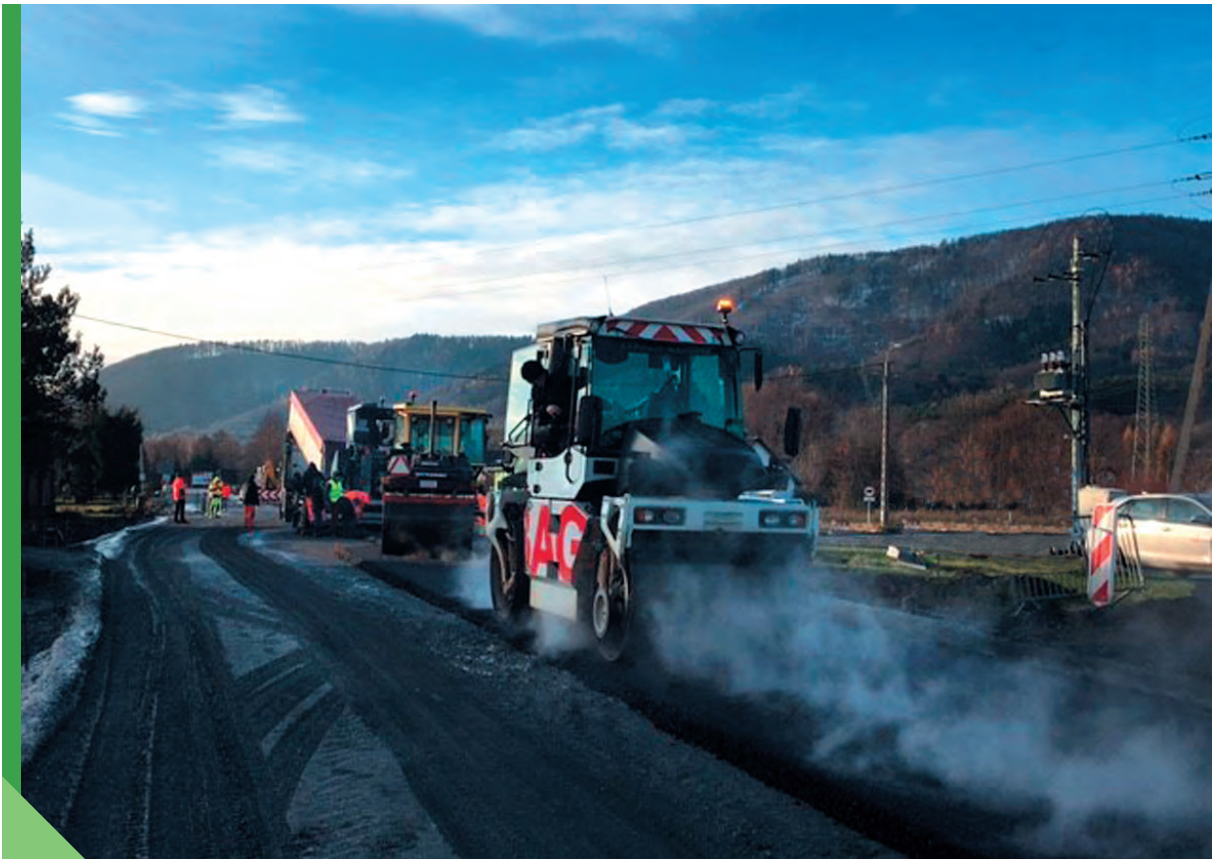
Fig. 3.17. Construction of an experimental road section using the ORBITON 45/80-80 HiMA WMA bitumen in 2021 [photo ORLEN Asfalt sp. z o.o.]
