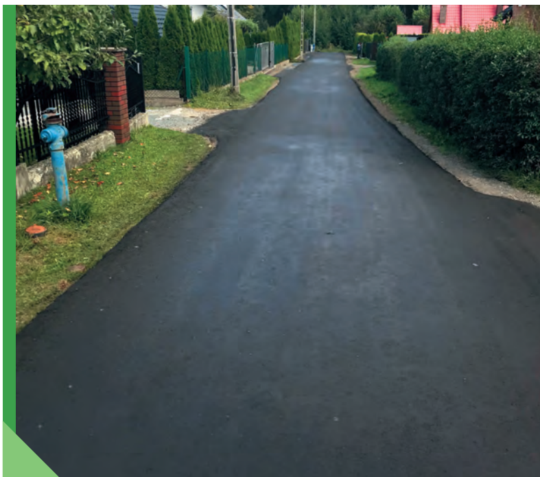
Fig. 5.5. Ready-made course made of GE mix (photo Eurovia Polska S.A.)
