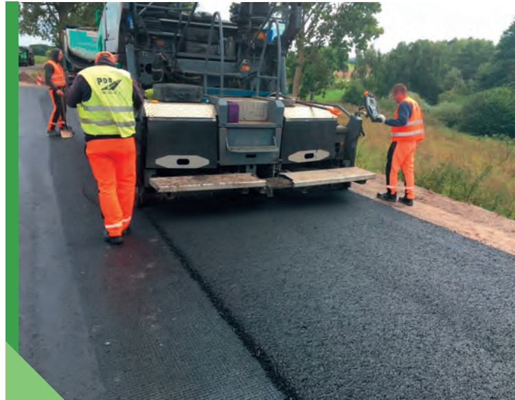
Fig.3.8. Experimental road section with bitumen 35/50 WMA constructed in 2021; measurement of the binder course temperature behind a spreader [photo K. Niemyjski, ORLEN S.A.]
