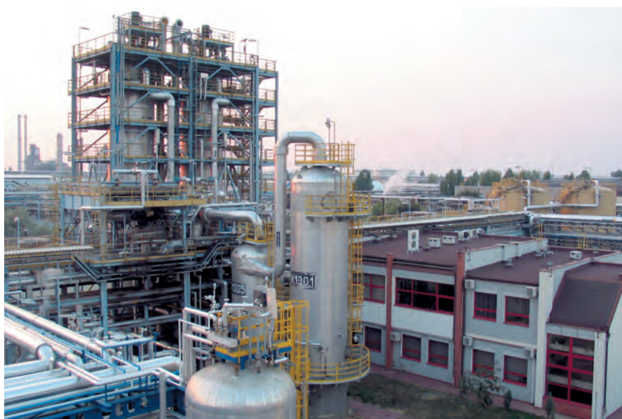
Fig. 1.3. Continuous oxidation system – Biturox® reactors (photo by ORLEN Asphalt)
